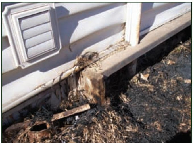
The homeowner stated that wind shifts from west to north brought the fire to the house. The fire department initially started suppression. Observations noted fire brands being carried by the wind to the side of the house and dropping them into the grass. Grass growing up under vinyl siding ignited, and consequently, the heat began to melt the siding and ignited the lattice on the back of the home.
