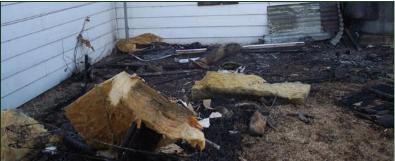
Despite numerous spot fires observed around the front of the home, ignitions actually occurred on the backside of the home. The large amounts of debris within close proximity to the home are credited with contributing to the ignition of the home.
